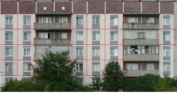
Figure 12: Starting another additional grid.
